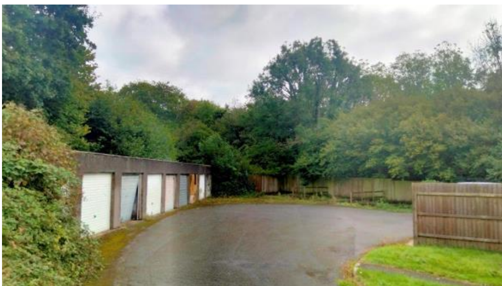
FIGURE 16: APPLICATION SITE PHOTO TAKEN FROM THE GREEN INFRASTRUCTURE STATEMENT
