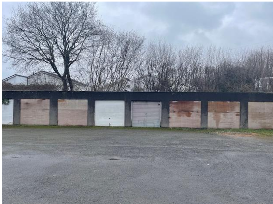
FIGURE 12: GARAGES TO BE DEMOLISHED
